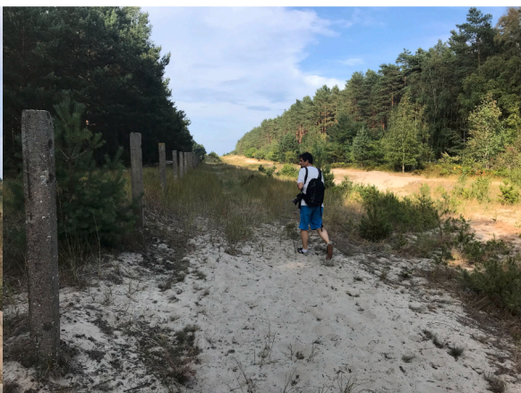
Figure 4d. Original border fence falling into dereliction
